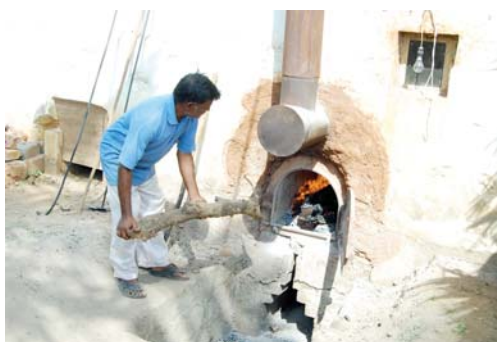
Venturi furnace to reduce the fuel usage
